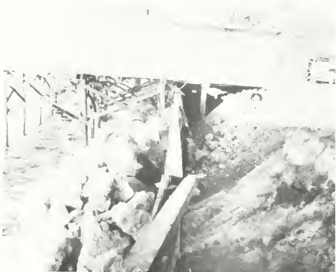
FIGURE 131.—Detail of the breaching of the seawall at Malibu Beach, Calif., by the perigean spring tides of 1974 January 8. The deep cavitation behind the wall is produced by erosional action resulting from the overspilling seas.
